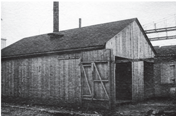
Figure 10. Fumigation Building at Key West Florida. 10
